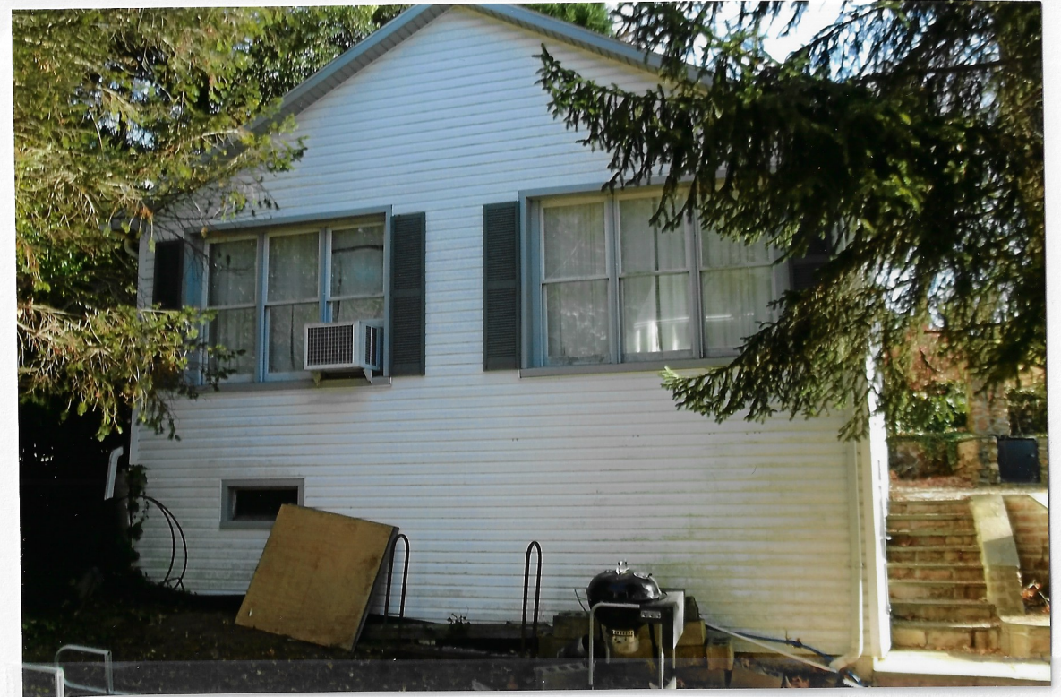
WEST SIDE OF EXISTING DWELLING
