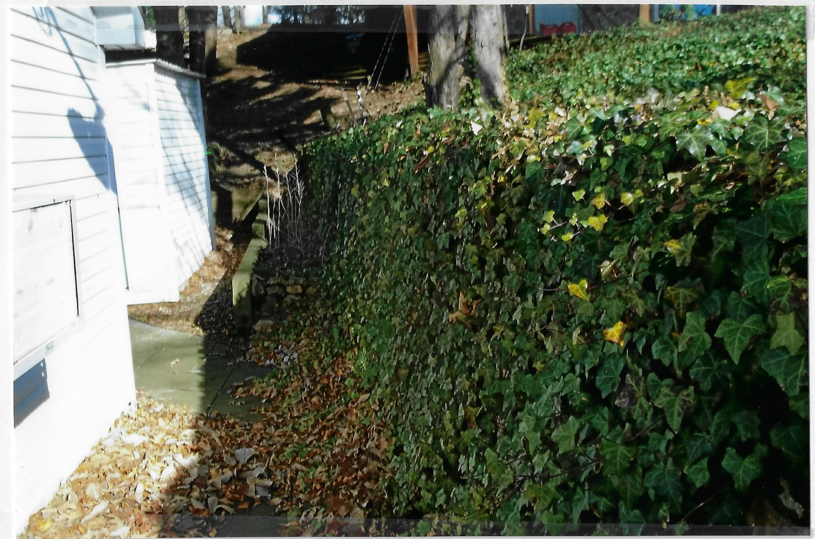
EAST SIDE OF EXISTING DWELLING AND STONE RETAINING WALL
