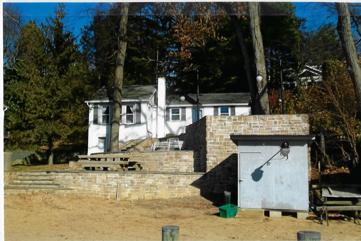
VIEW FROM WATER LOOKING TOWARDS ROAD
