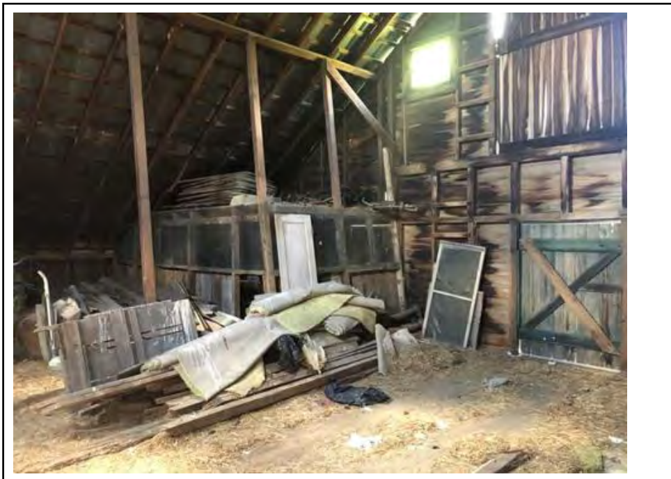
INTERIOR OF BARN OF SUBJECT PROPERTY
