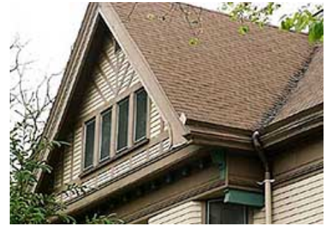
Gable End Profile Trim, Gutter and Downspout Examples
