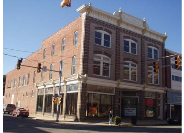
Commercial Window and Façade Examples
