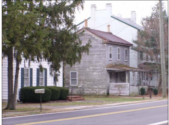
This house at 11947 Augustine Herman Highway is one of several deteriorated structures in the village. The “Groves House” located in the background is listed on the Maryland Inventory of Historic Places.
