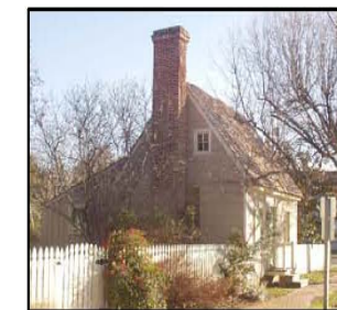
HISTORIC COTTAGE ELEVATION FROM STREET
