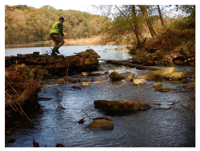
Figure 4. Rubble and cement at breach in earthen dam looking upstream toward Mill Pond
